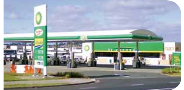
BP Connect Rosedale, Albany. Site on completion of upgrade in March 2010.
